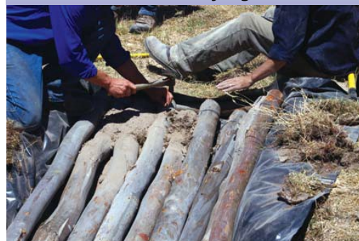
Wiring in the logs
