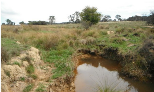
Headcut threatening an intact floodplain. If left unchecked, a gully will form through the valley floor which will ultimately dehydrate the surrounding landscape
