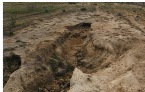
A rill beside a farm road. Works can stabilise and stop further damage to infrastructure.
