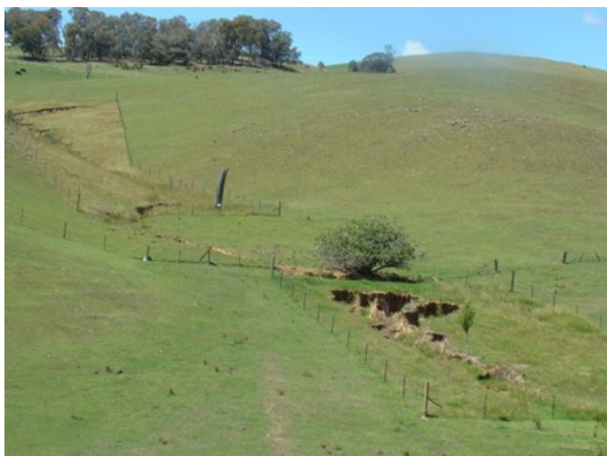
The gully area after it has been fenced off, to control stock access
